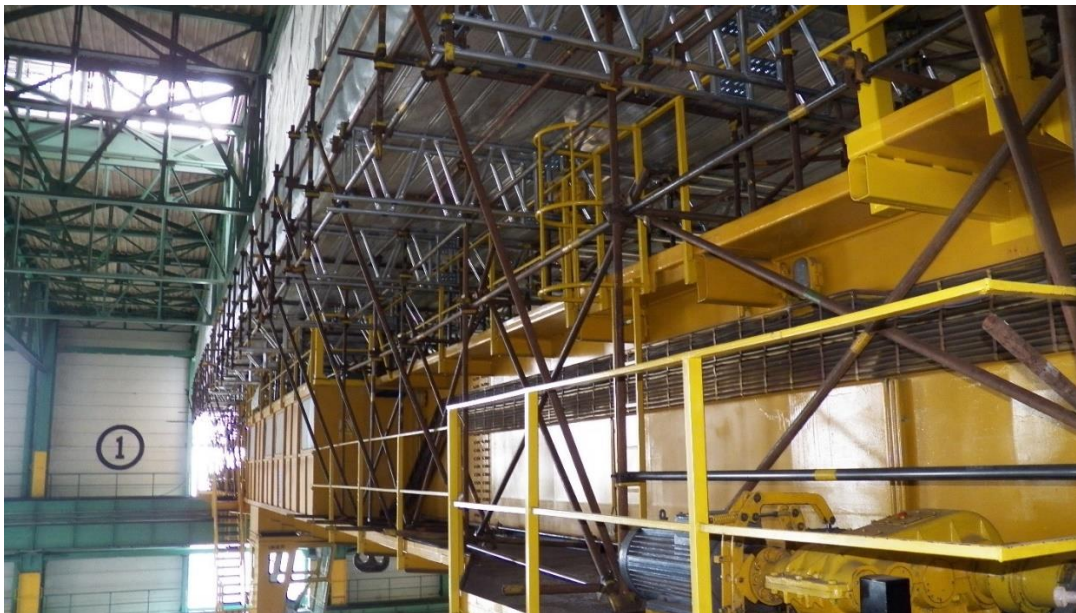
Figure 6. Construction of a work platform on a crane bridge
