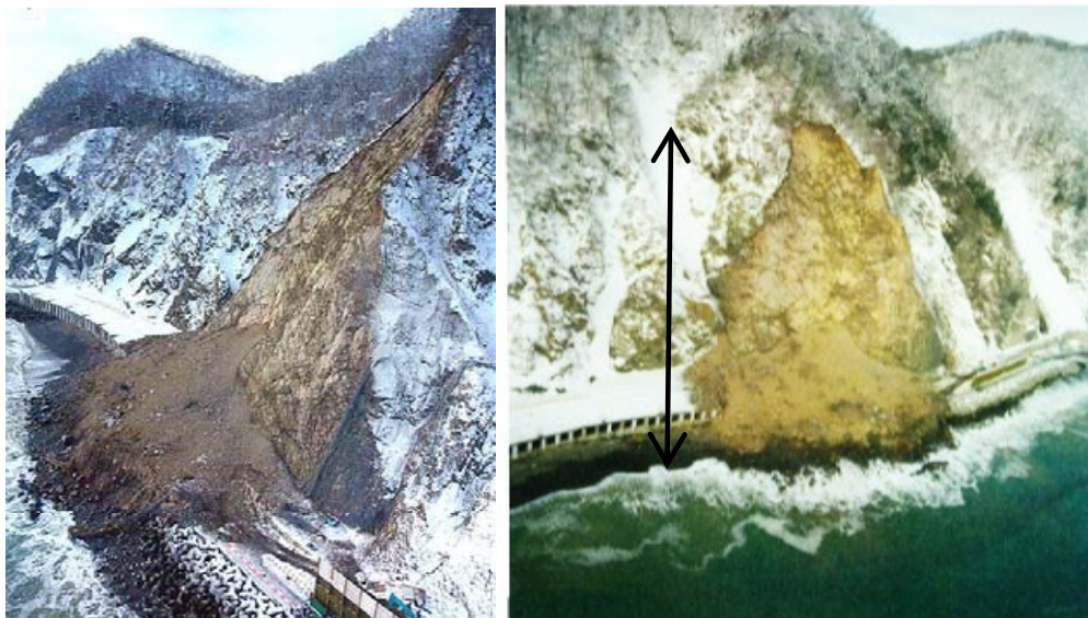
Figure 1. Bedrock collapse of Erimo-cho in 2004
