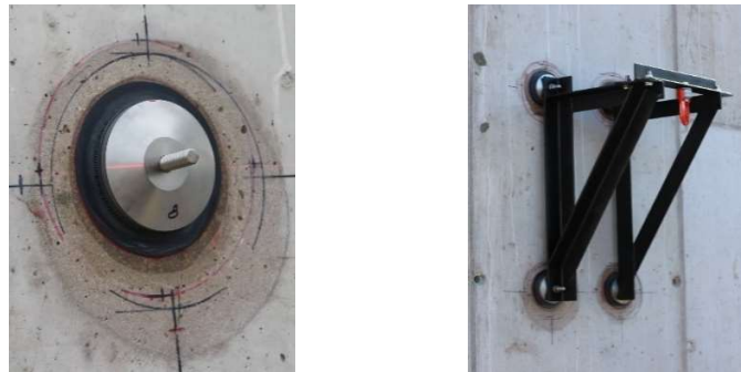
Figure 6. Left: C-BLOCK bonding on concrete – Right: lifting frame installed with 4 C-BLOCKS
