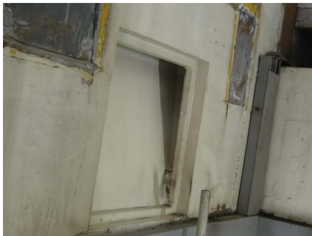
Figure 8. Openings in the concrete and previously installed steel plates
