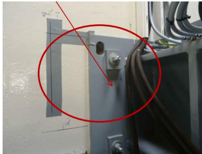
Figure 6. Back side of the through-wall-anchor in the neighboring room
