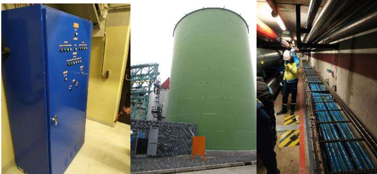
Figure 8: Illustration of post-earthquake plant walkdown.
