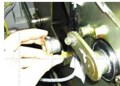
Fig.8 Damage of circuit breaker
