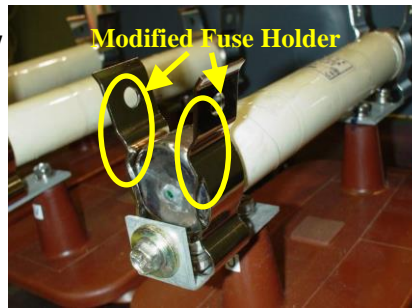
Fig.7 Modified fuse holder
