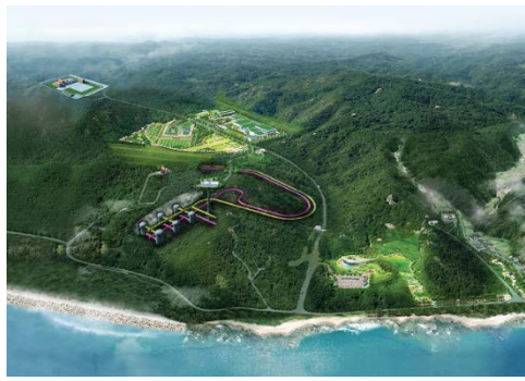
Figure 1. LILW disposal facility in Wolseong
