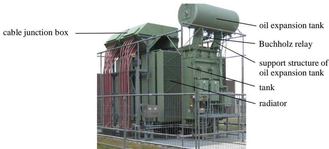
Figure 2. 110 kV-plant feeding transformer (original configuration without structural improvements)
