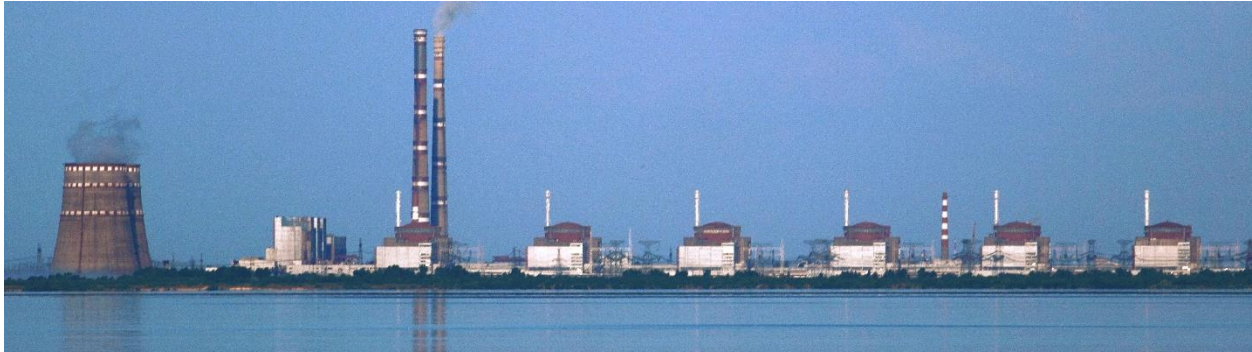
Figure 5: Zaporizhzhia NPP, the two cooling towers and the 6 VVER reactor buildings (Ralf 2009)
