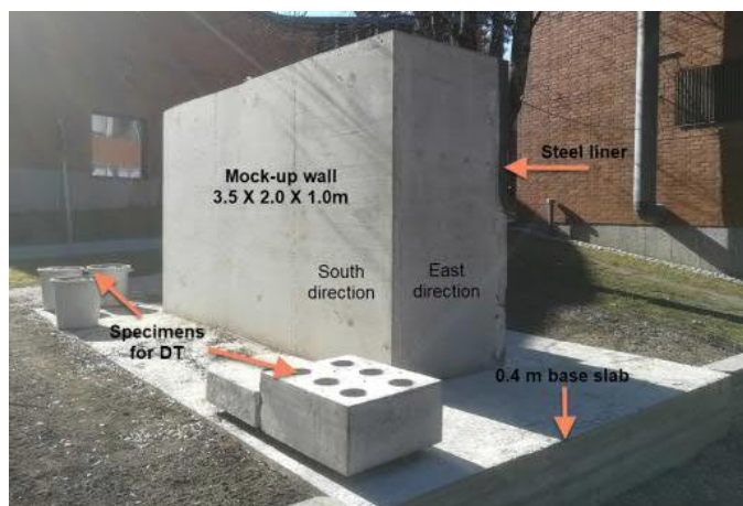
Figure 1 – Overview of the thick-walled concrete structure (Al-Neshawy et. al., 2018).
