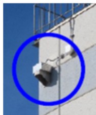
(a) Accelerometer on exterior walls
