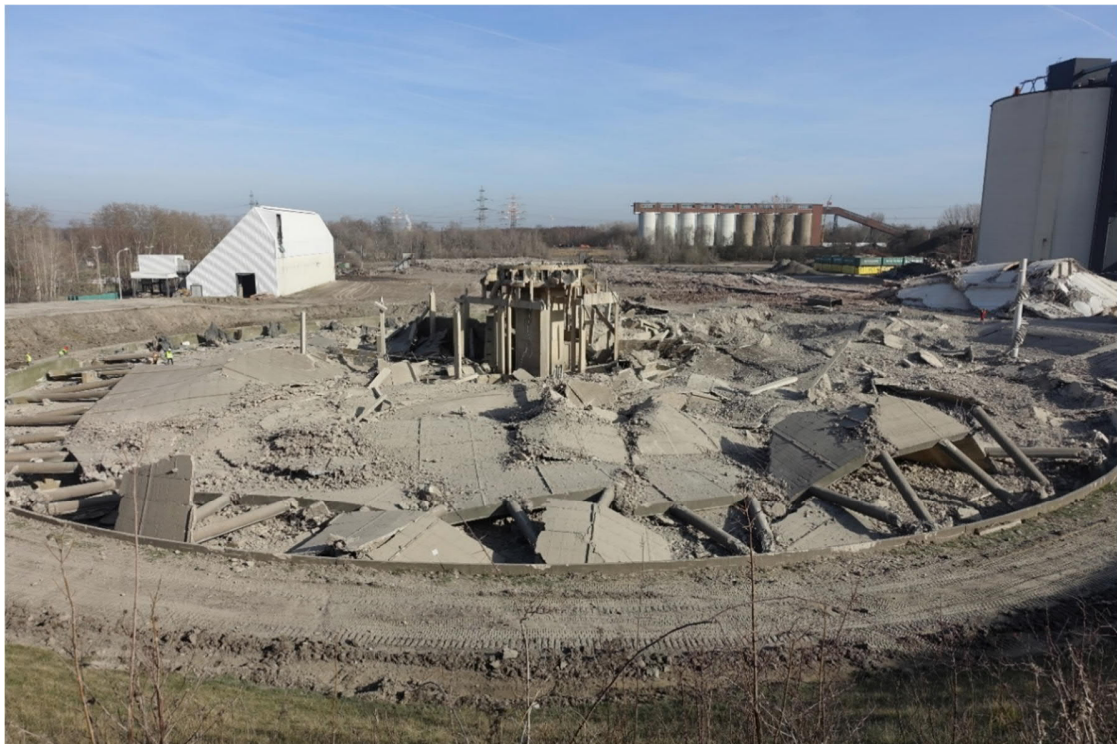
Figure 7: Cooling tower in Knepper (Germany) power station after the blasting
