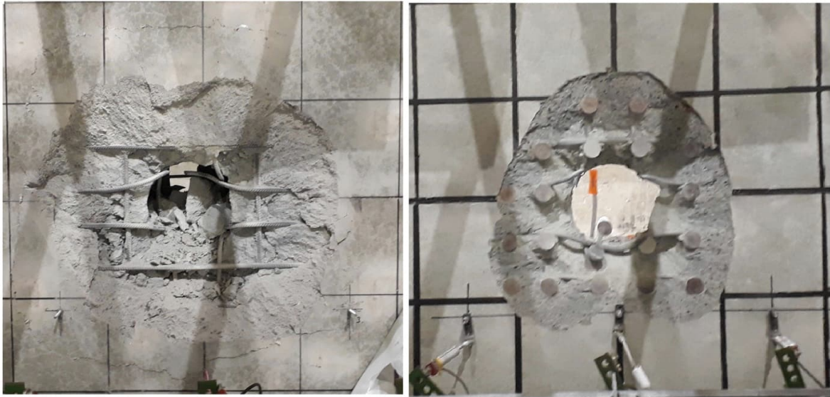
Figure 6. Front surface of slabs ITP2RR (left) and ITP4RR (right) after the test.
