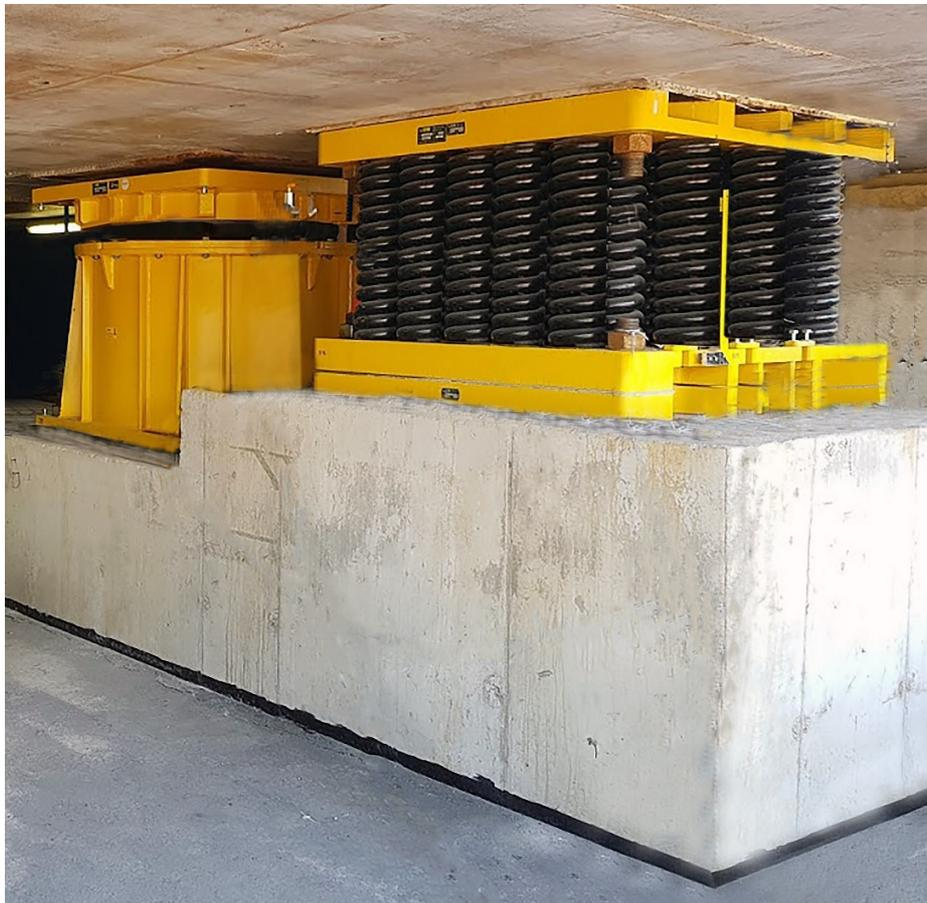
Figure 1. Viscous damper (left) and spring element (right) below concrete superstructure.
