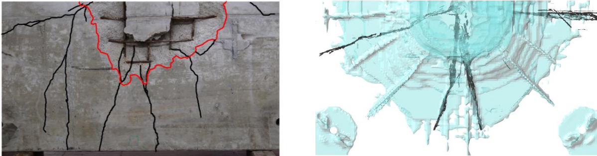
Figure 5. Combination of damage characterizing information; at left cracks and scabbing on the back of half plate # P300; at right superposition of the crack structures from tomography and FEM
