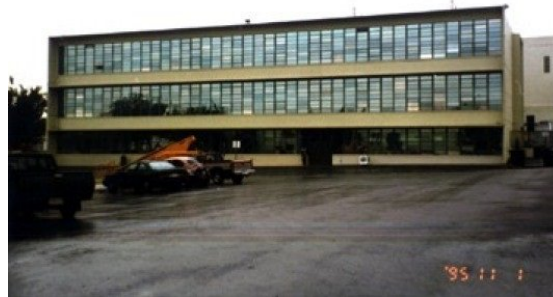
CGS CSMIP-35409 Taft - 3-story School Bldg.
