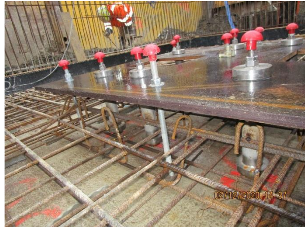
Figure 2. Illustration of anchorages with T-head bolts
