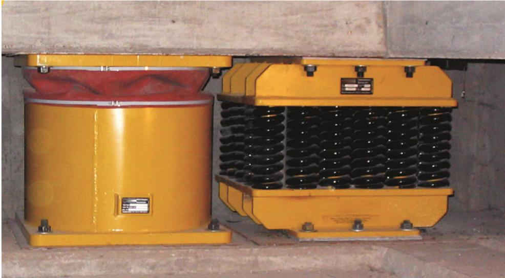
Figure 1. Viscous damper (left) and spring element (right) below concrete building
